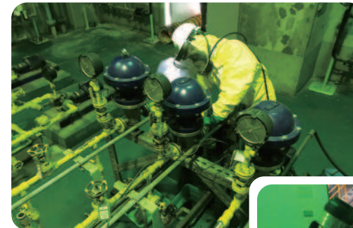
Emergency response drill for chemical (ammonia) spills
