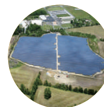
Ground-mounted/Lumberton Solar Plant, New Jersey,
