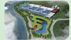
Zhongli Wastewater Sewage System (BOT)
