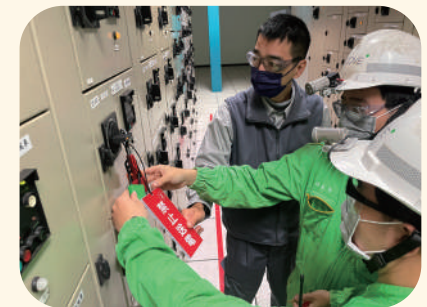
Joint confirmation by operation, maintenance, and HSE personnel
