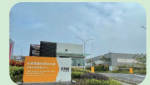
TSMC Reclaimed Water Plant at Southern Taiwan Science Park
