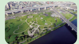
New Taipei City Gravel Contact Oxidation Treatment and Water Resource Center
