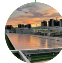
Roof-mounted/Taichung Metro/5.6 MWp
