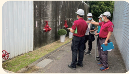
Fire Brigade Supervision and Inspection Operation - Compliance with Regulations
