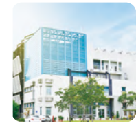
Tainan Science Park Plant
