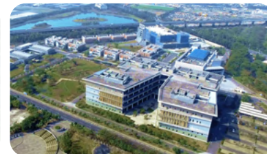
Water Treatment Plant of Pingtung Agricultural Biotechnology Park
