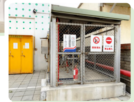
Replacement of heavy oil with natural gas.
