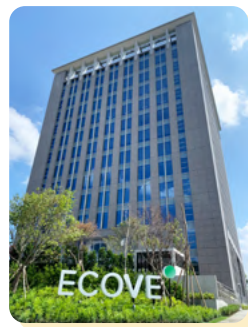
ECOVE's headquarters won the EEWB Green Building Label - Diamond and Smart Building Label - Diamond.
