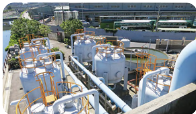
Zhonggang Water Resource Center
