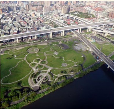
New Taipei City Gravel Water Treatment Plant
