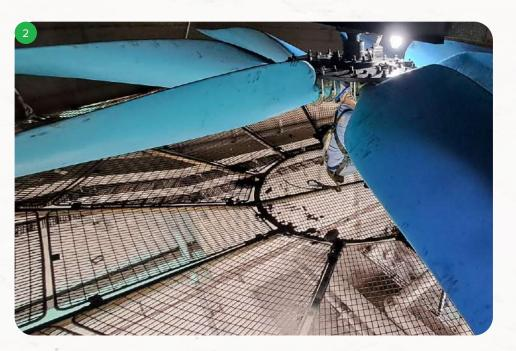
2 Replacement of ACC fans with Fiberglass Reinforced Plastic (FRP) blades and other modifications
