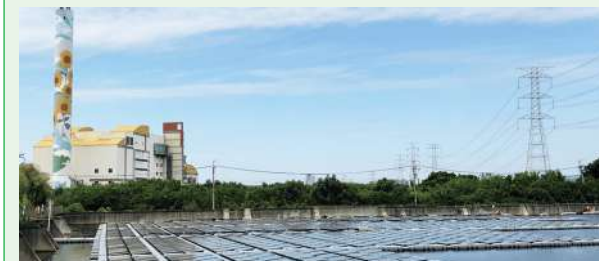
Floating/High-Speed Rail Wurih detention basin/0.3 MWp
