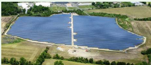
Ground-mounted/Lumberton Photovoltaic Power Plant, New Jersey, USA/9.5 MWp
