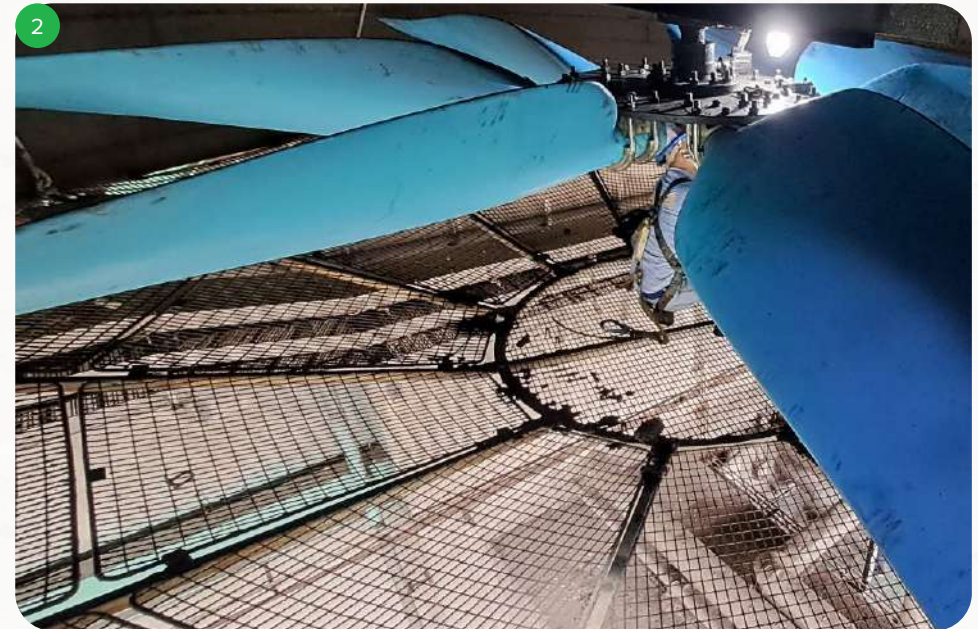
2 Replacement of ACC fans with Fiberglass Reinforced Plastic (FRP) blades and other modifications
